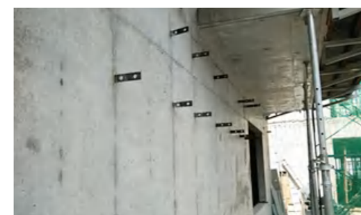
Aluminium Formwork Forming Effect
