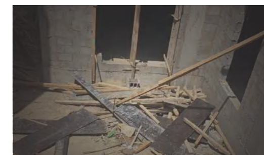
Timber Formwork on Site
