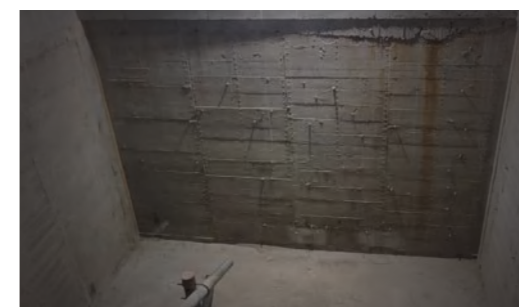
Timber Formwork Forming Effect
