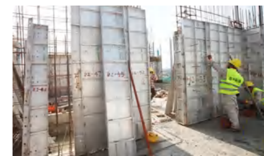
Aluminium Formwork on Site
