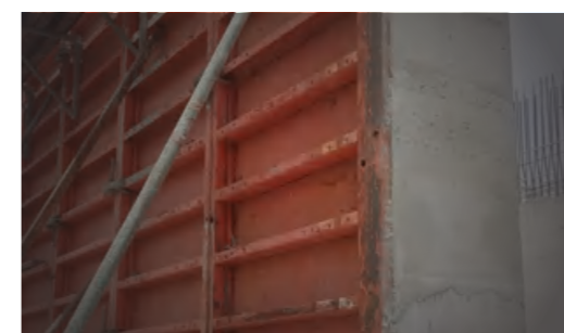
Steel Formwork Forming Effect
